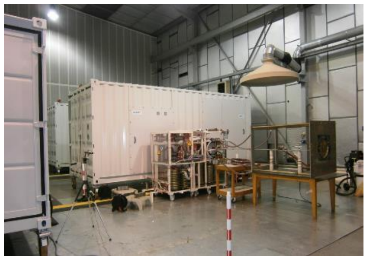
Commissioning and SAT on customer test room
